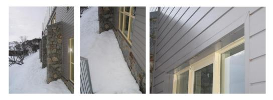
We have recently been working through the Bushfire Hazard Assessment and to achieve the required Bushfire Attack Level of BAL 40 we need to remove all the existing high maintenance and potentially flammable external timber wall cladding and replace with Colourbond Steel Cladding to improve the aesthetics of the building and reduce the fire damage risk at the same time.
